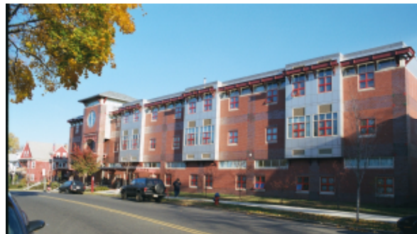
West Somerville Neighborhood School Somerville, MA
