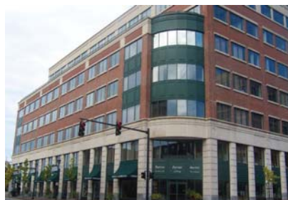
Two Portland Square Office Building Portland ME
