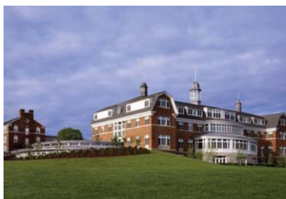
Salisbury School Library/Humanities & Arts Buildings Salisbury CT
