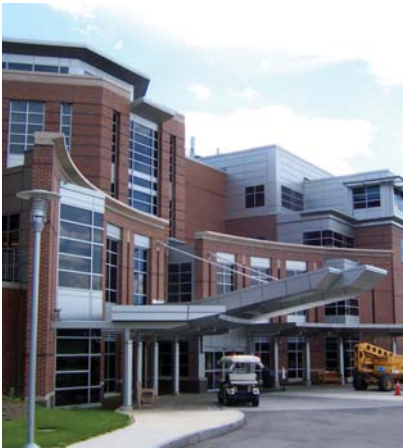
Concord Hospital Addition Concord NH
